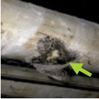
Asbestos sheets
