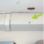
Asbestos cardboards
