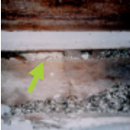
Grains containing asbestos used for insulation
