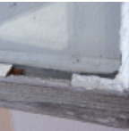
Highly weathered window putty
