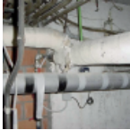
Sprayed asbestos for insulation
