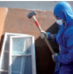
Knocking out glass with a hammer (outdoors)
