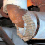
Damaged pipe insulation
