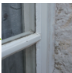
Caulking between window masonry
