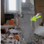
Cement-bound heating pipes
