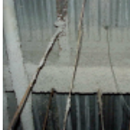
Sprayed asbestos for fire protection
