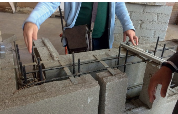
Hemp and lime-based blockwork at CEFME-CTP training centre
