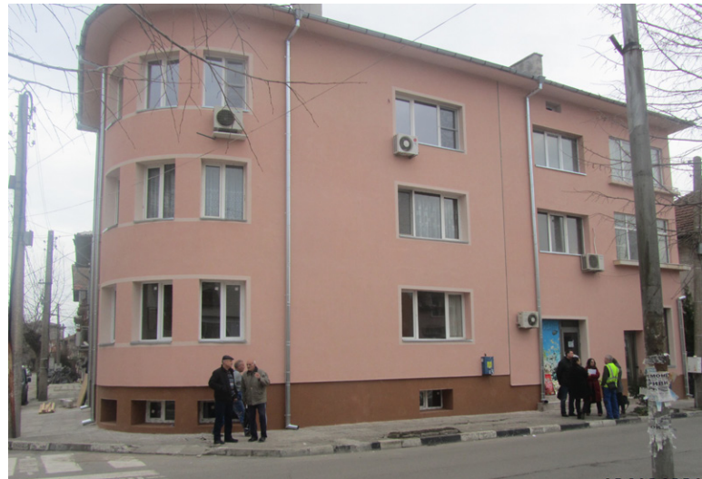
Retrofitting project in Mazdra
