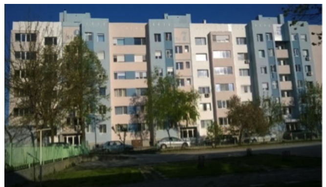
CASE STUDY 2: Multifamily residential building (Silistra) – Before and after renovation
