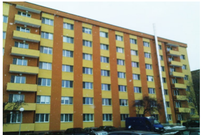
CASE STUDY 1: Military social housing 'MAY' (Sofia) – Before and after renovation
