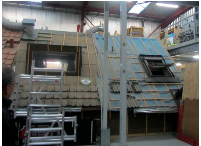
Mock-up of roofing insulation: CDR Training Centre, Brussels
