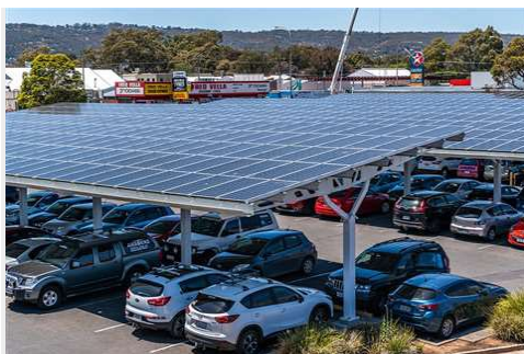
A car park with solar PV panels mounted on solar shades (Image: Wikimedia Commons)
