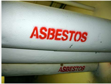
Asbestos pipe lagging (Image: daryl_mitchell/Wikimedia Commons)
