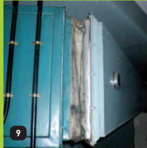
Insulation for pipe ducts against fire, heat and cold
