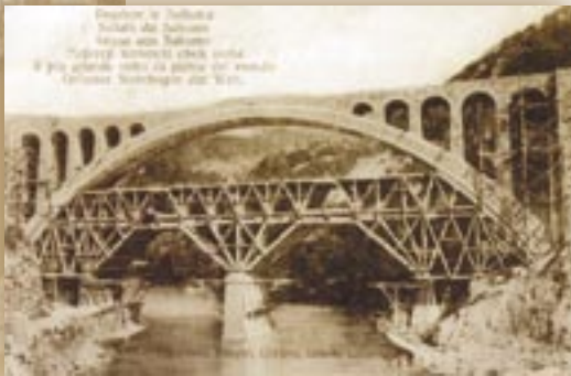
Stone Railway Bridge, Solkan, Slovenia, 1904-1906 (Line Vienna-Trieste, largest stone arch in natural stone in the world, 85 m span, 5,000 tonnes of stone, construction time 18 days)
