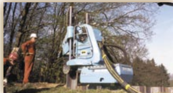
Driving sheet steel piles
