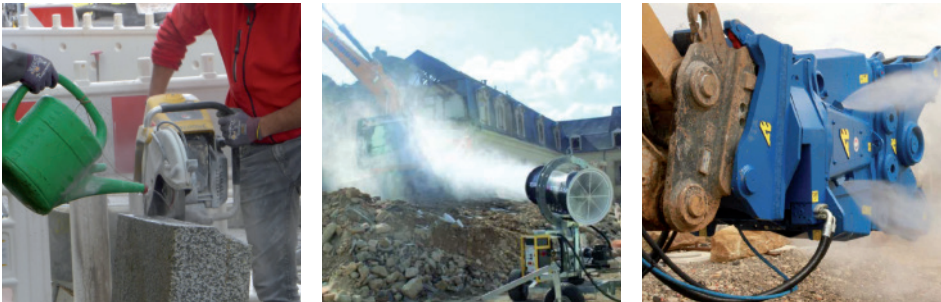
FIGURE 8: Dust binding by water
