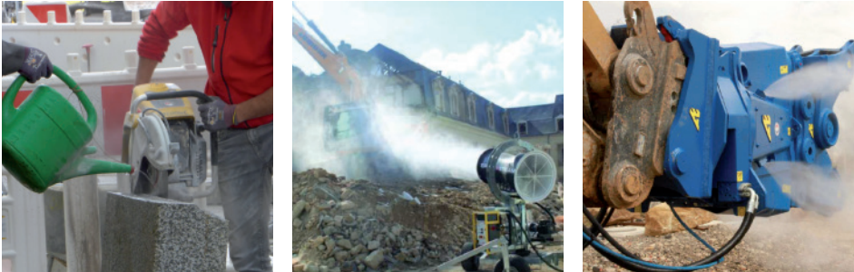
FIGURE 8: Dust binding by water
