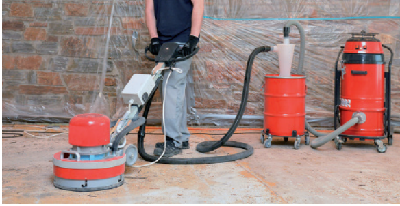
FIGURE 17: Pre-separator (centre) and vacuum cleaner (right) when using a floor sanding machine
