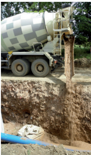
FIGURE 20: Liquid soil is filled into a trench
