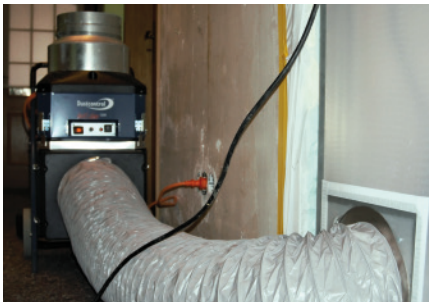
FIGURE 15: Air cleaner on construction site
