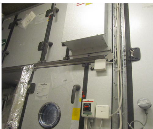
Metsatammi heat recovery and mechanical ventilation system
